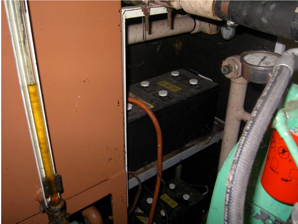
Picture 30 – Unit 4 CUL 280 Engine Start Battery
