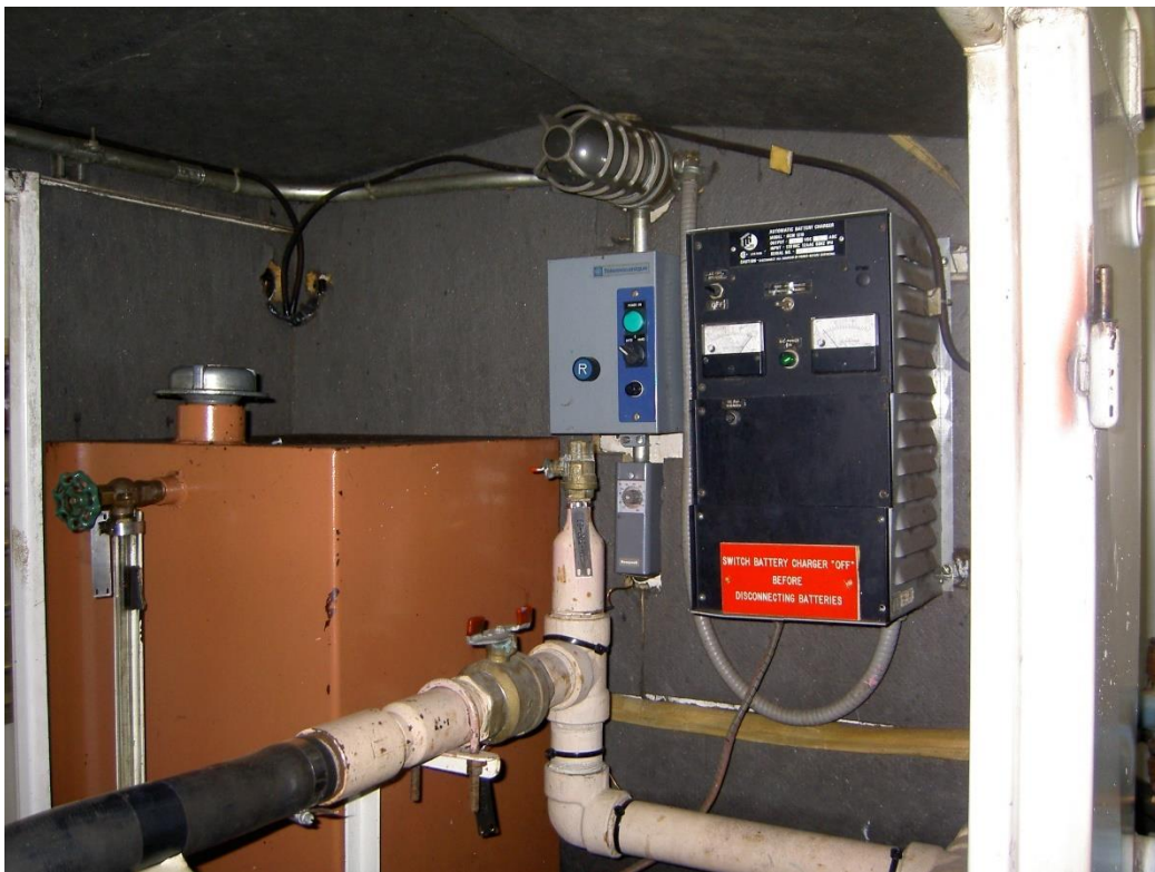
Picture 31 – Unit 4 CUL 280 Engine Battery Charger
