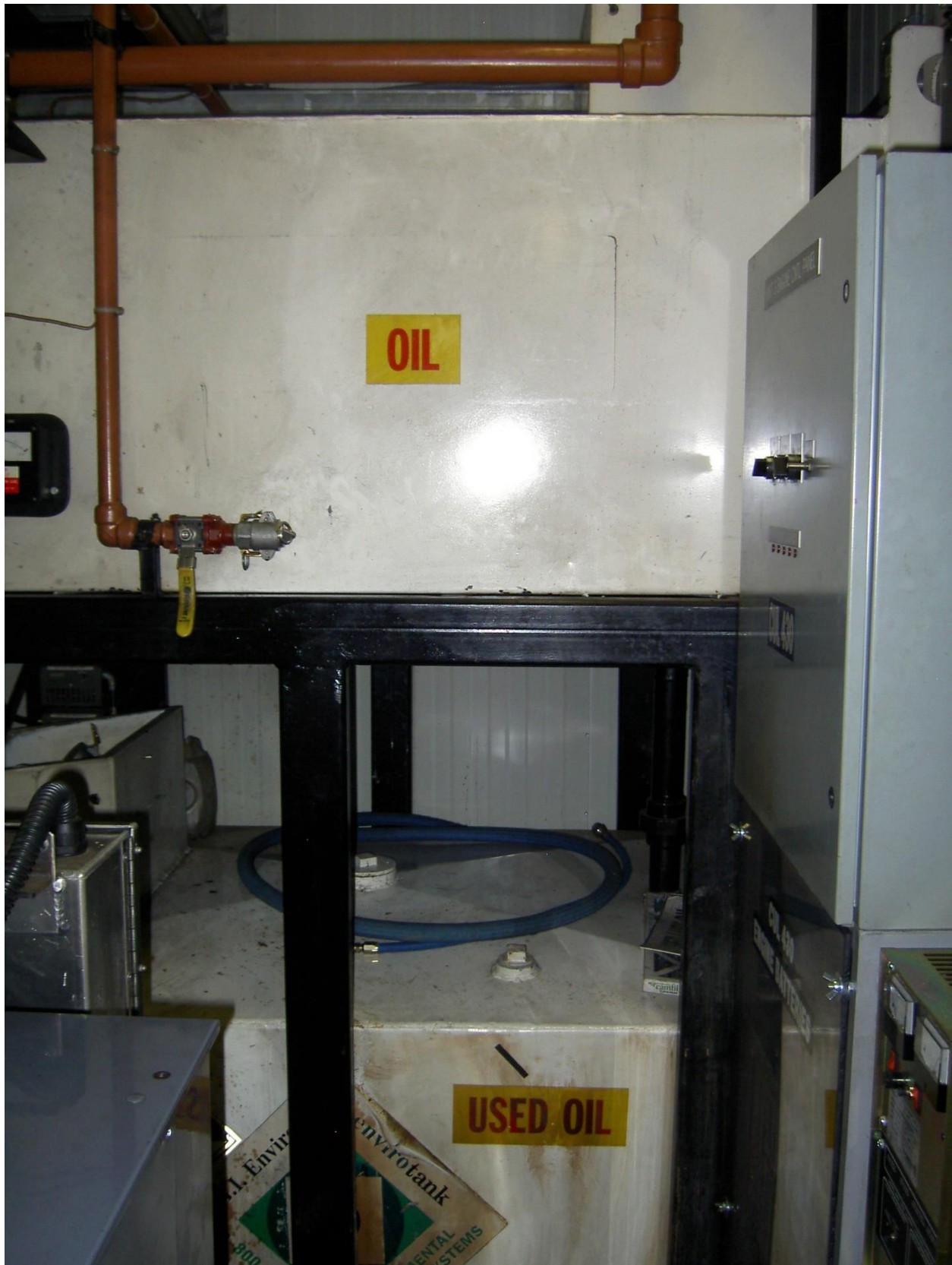
Picture 11 – New and Used Oil Tank in Generator Building
