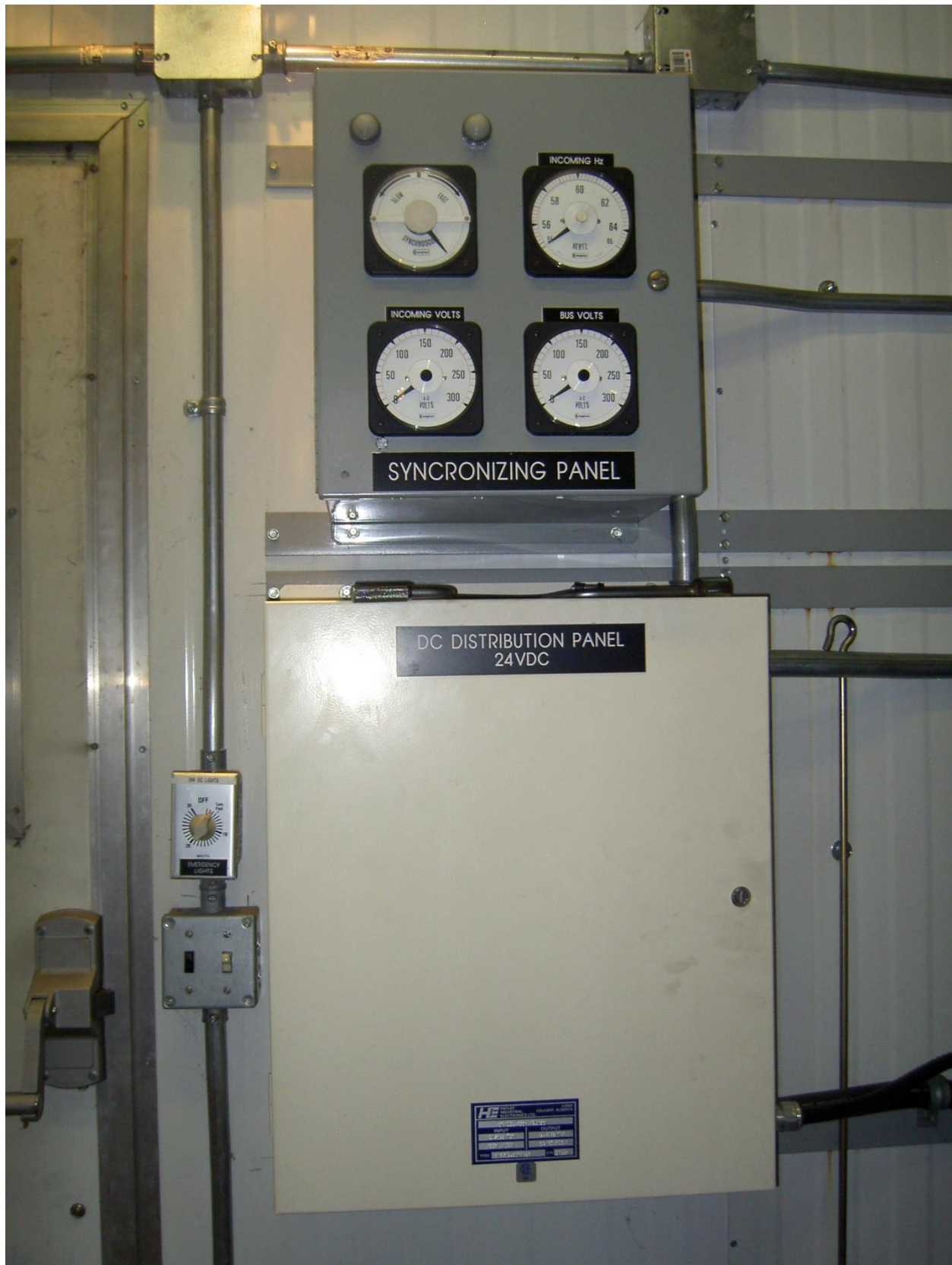
Picture 5 – Synchronizing Panel
