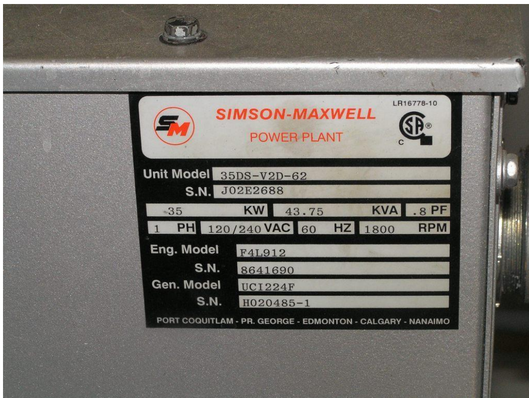
Picture 16 – Unit 2 CUL 429 Generating Unit Nameplate
