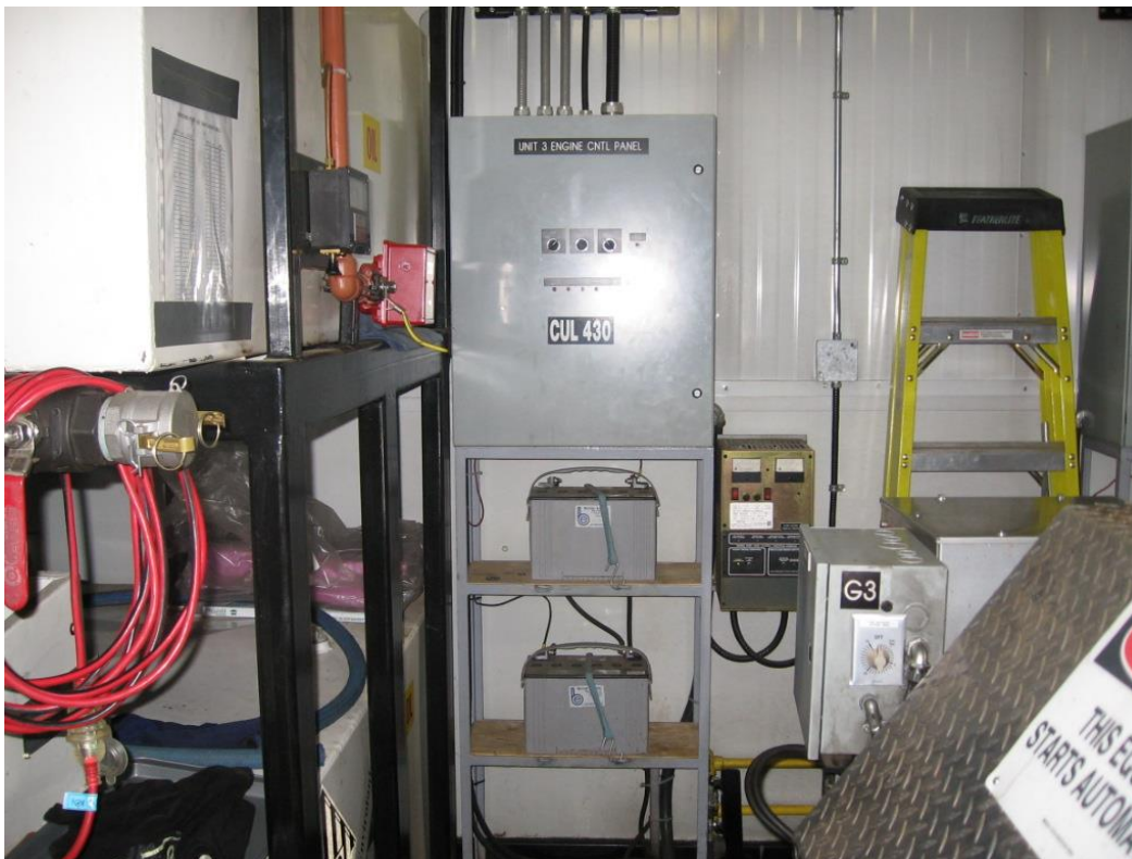
Picture 20 – Unit 3 CUL 430 Engine Control Panel, Start Battery and Battery Charger
