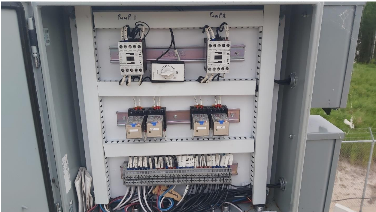
Picture 38 – 75,000 Litres Diesel Fuel Storage Tank 2 Pump Control Panel
