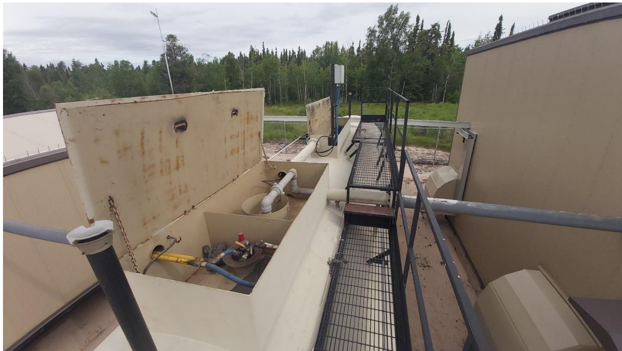
Picture 34 – 75,000 Litres Diesel Fuel Storage Tank 1 Spill Box and Walkway
