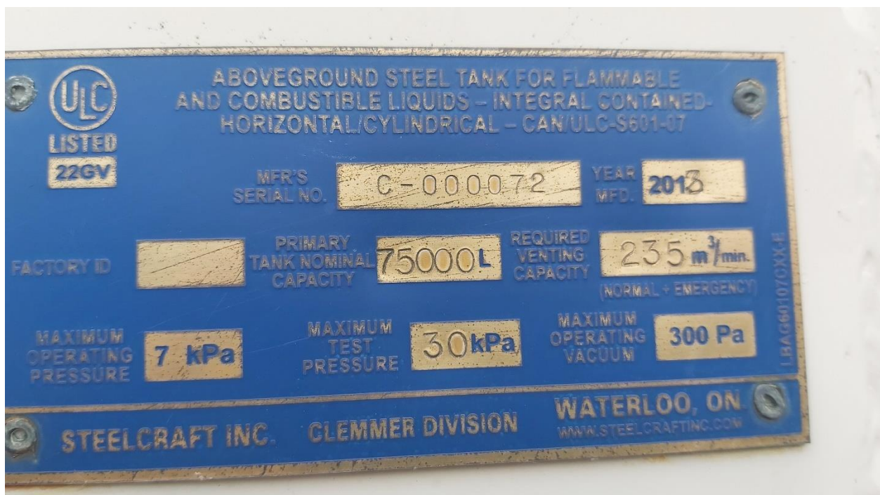
Picture 36 – 75,000 Litres Diesel Fuel Storage Tank 2 Nameplate
