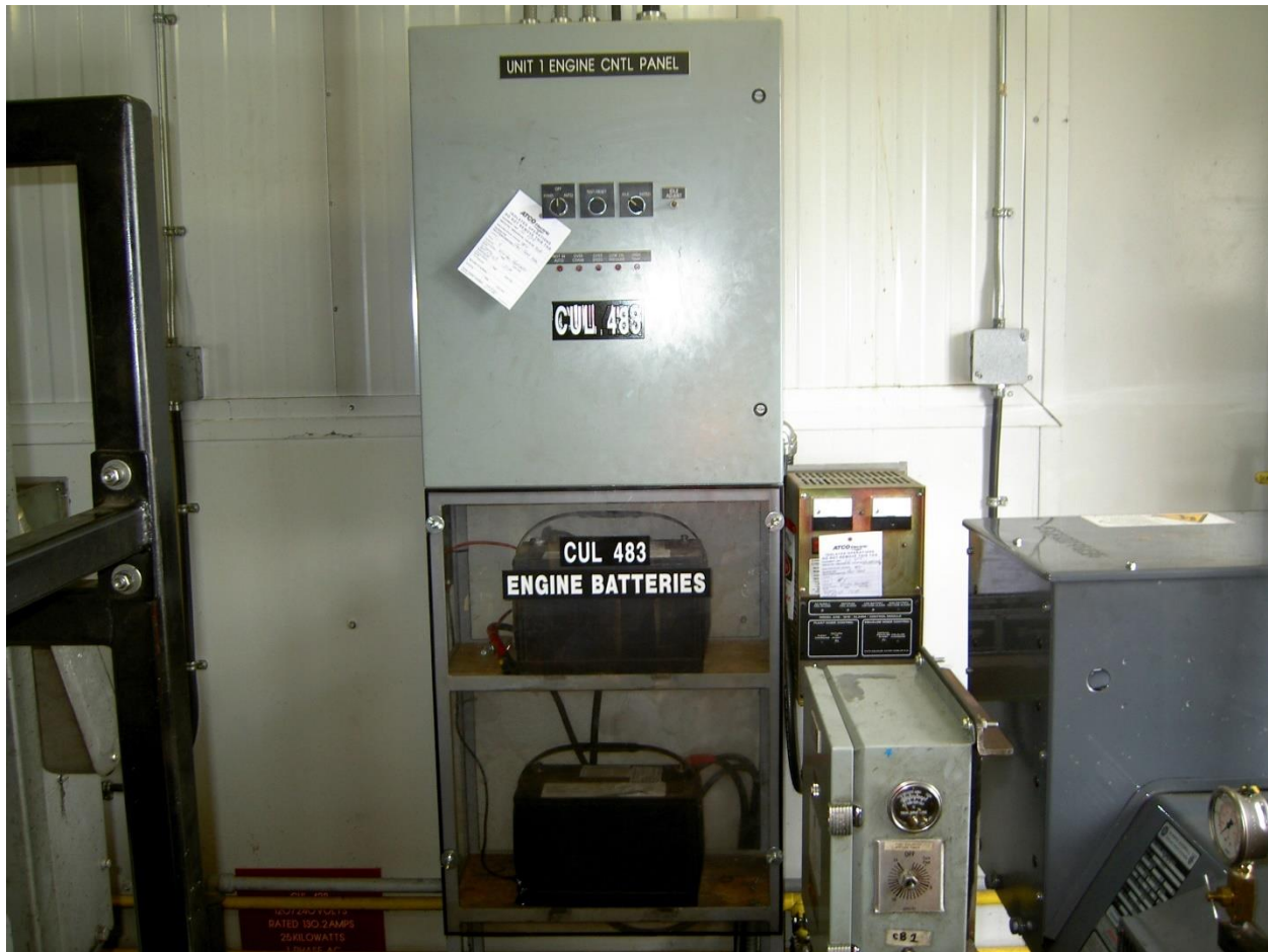
Picture 14 - Unit 1 CUL 483 Engine Control Panel, Start Battery and Battery Charger
