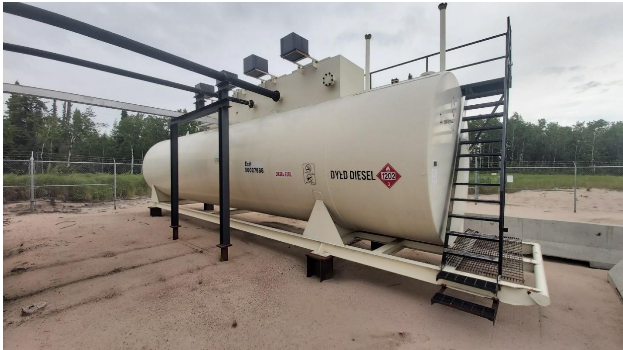
Picture 35 – 75,000 Litres Diesel Fuel Storage Tank 2
