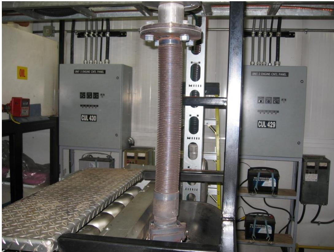
Picture 18 – Unit 2 CUL 429 Engine Control Panel, Start Battery and Battery Charger
