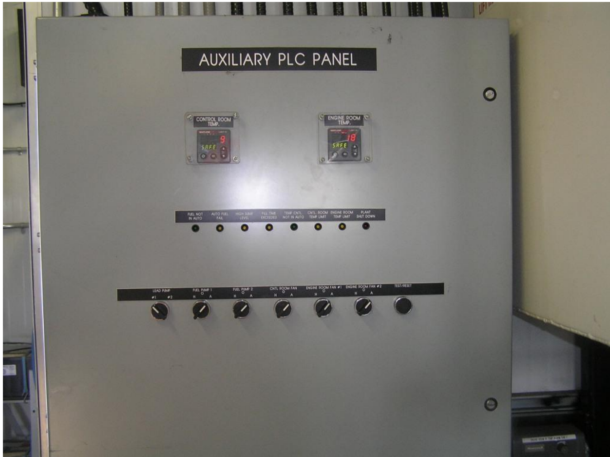
Picture 8 – Plant Auxiliary PLC Panel
