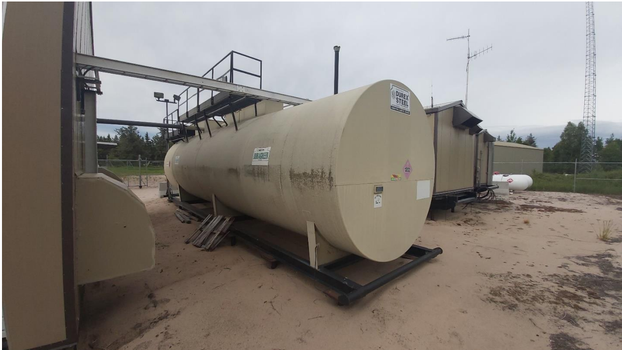
Picture 32 – 75,000 Litres Diesel Fuel Storage Tank 1
