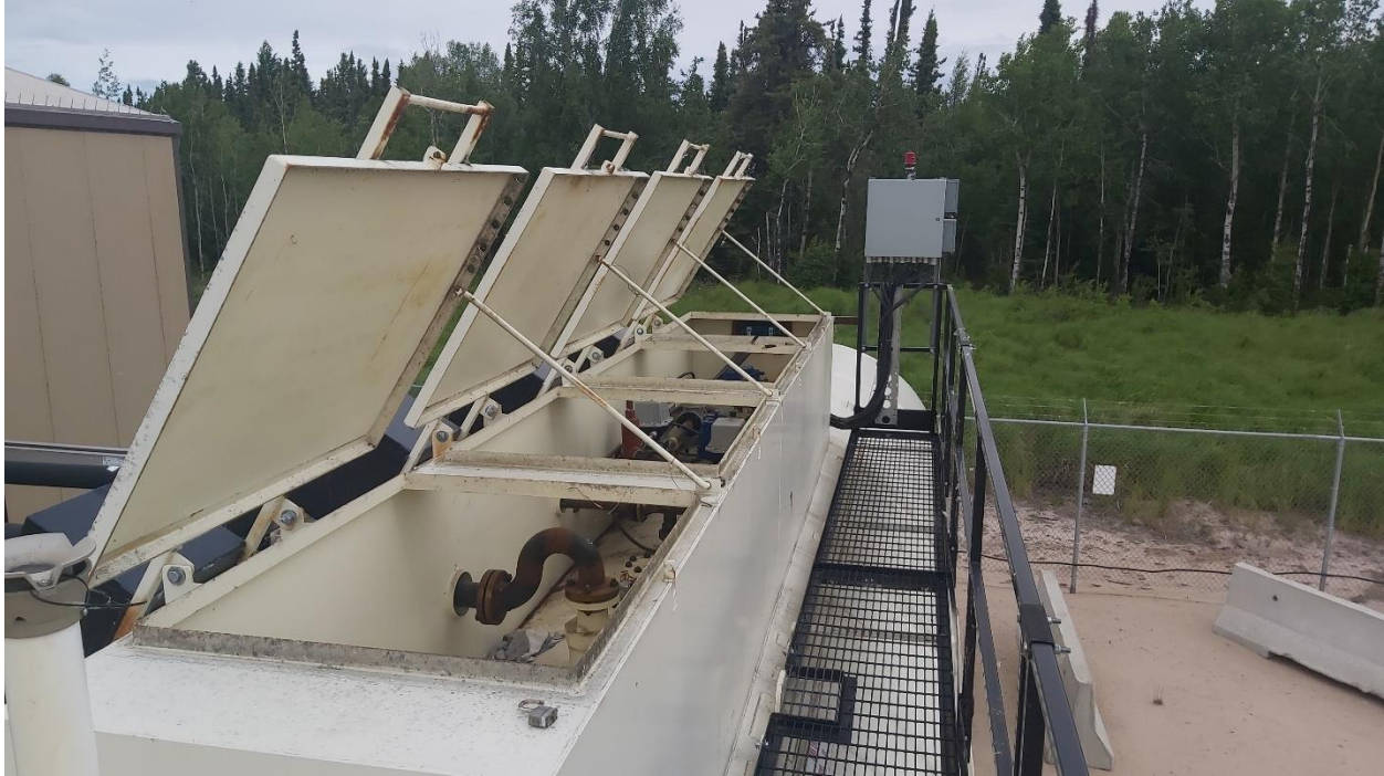
Picture 37 – 75,000 Litres Diesel Fuel Storage Tank 2 Spill Box and Walkway
