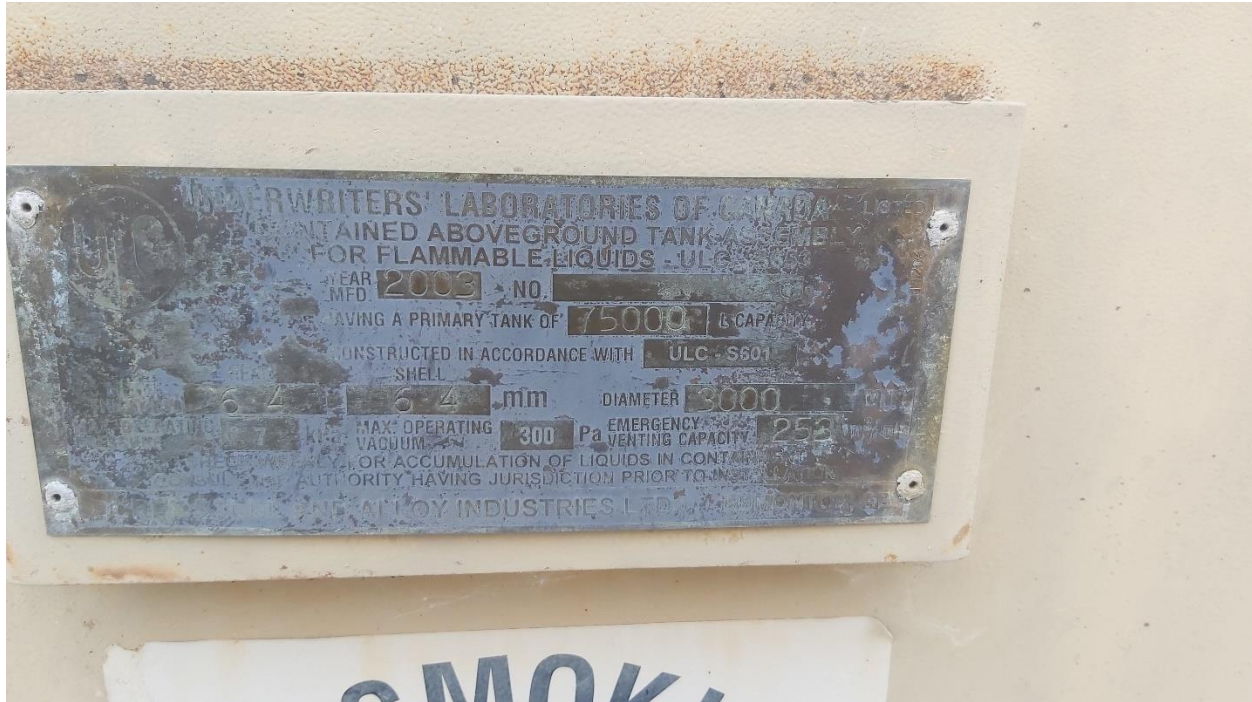
Picture 33 – 75,000 Litres Diesel Fuel Storage Tank 1 Nameplate
